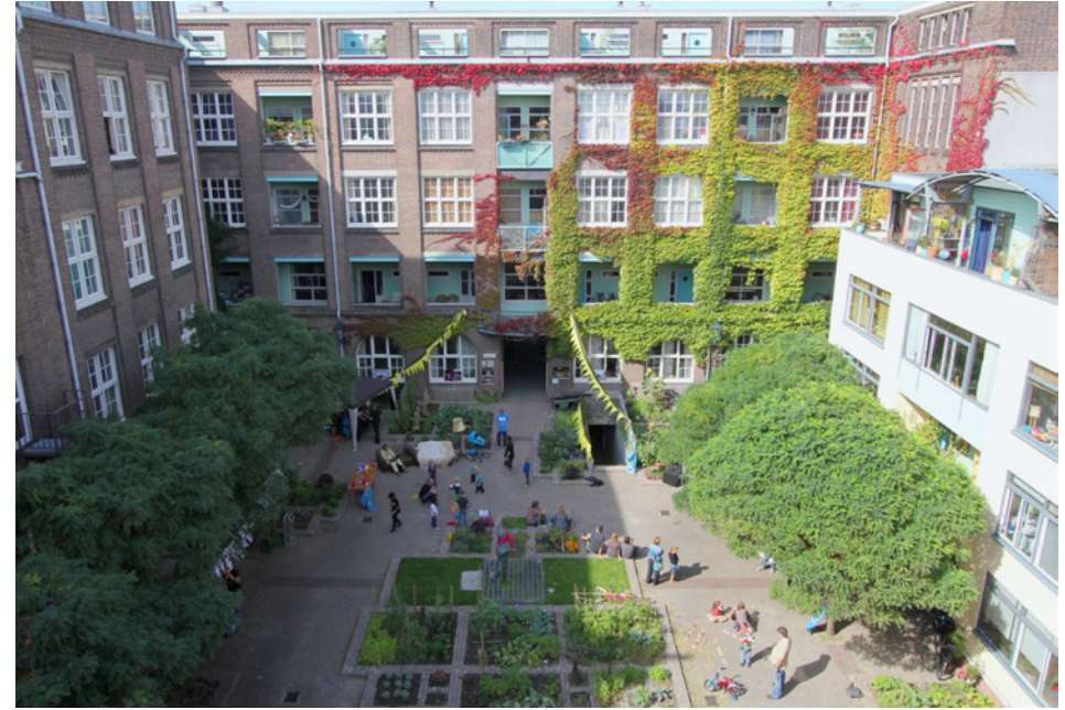
Fig. 1: Pander project, The Hague/the Netherlands, Scala Architects, 1985-1991
