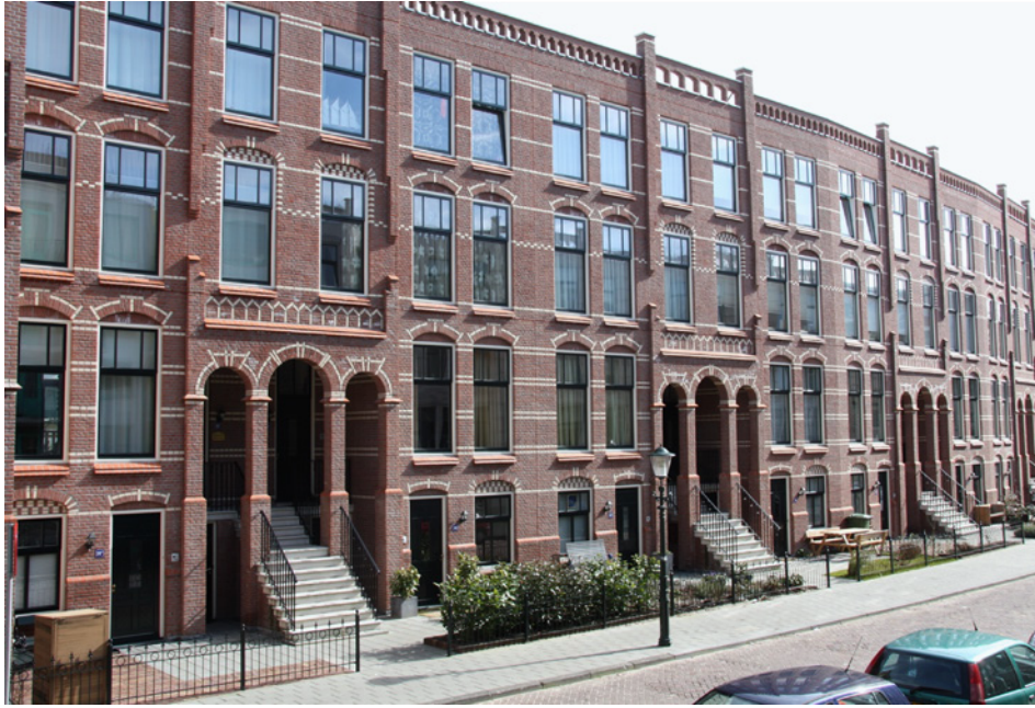
Fig. 2: Obrechtstraat, The Hague/the Netherlands, by Scala Architects, 2001–2008
