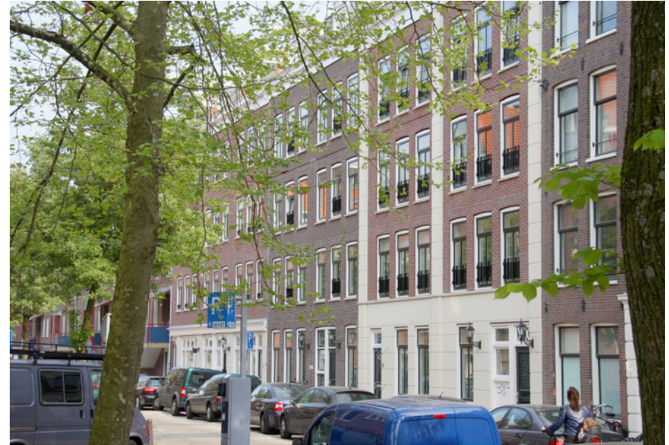
Fig. 5: Residential building, Barentszstraat, Amsterdam/the Netherlands, Scala Architects, 2010–2011
